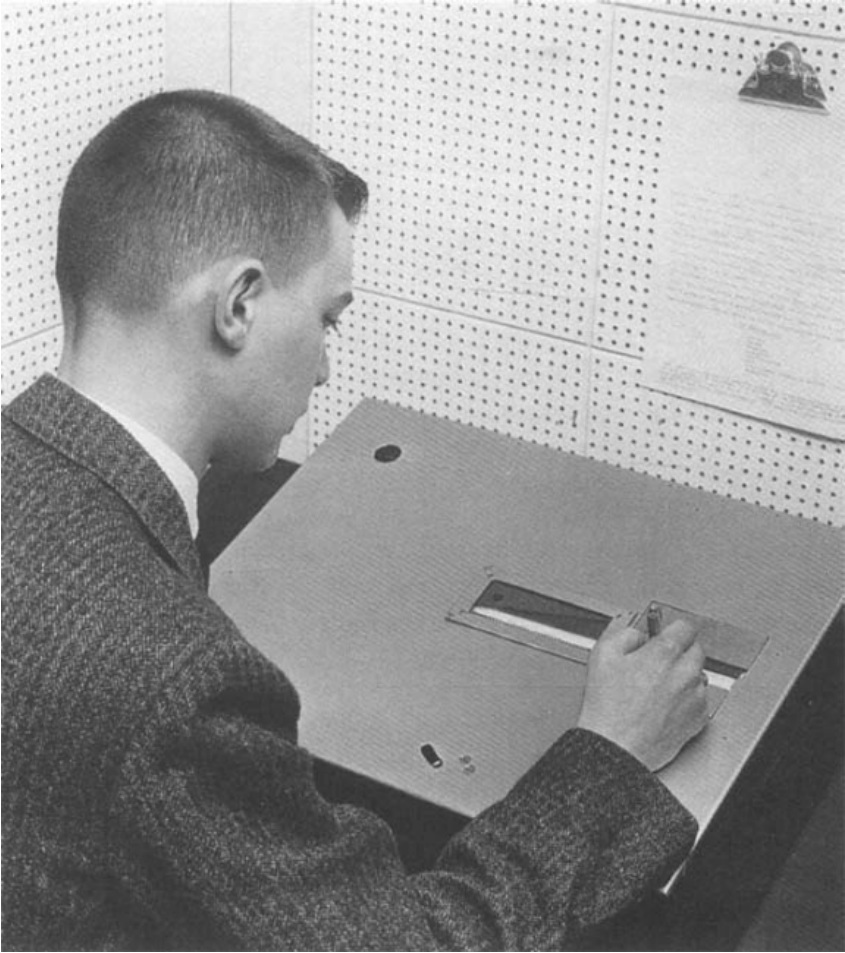
FIG. 2. Student at work in the self-instruction room. One frame of material is partly visible in the left-hand window. The student writes his response on a strip of paper exposed at the right. He then lifts a lever with his left hand, advancing his written response under a transparent cover and uncovering the correct response in the upper corner of the frame. If he is right, he moves the lever to the right, punching a hole alongside the response he has called right and altering the machine so that that frame will not appear again when he goes through the series a second time. A new frame appears when the lever is returned to its starting position.
