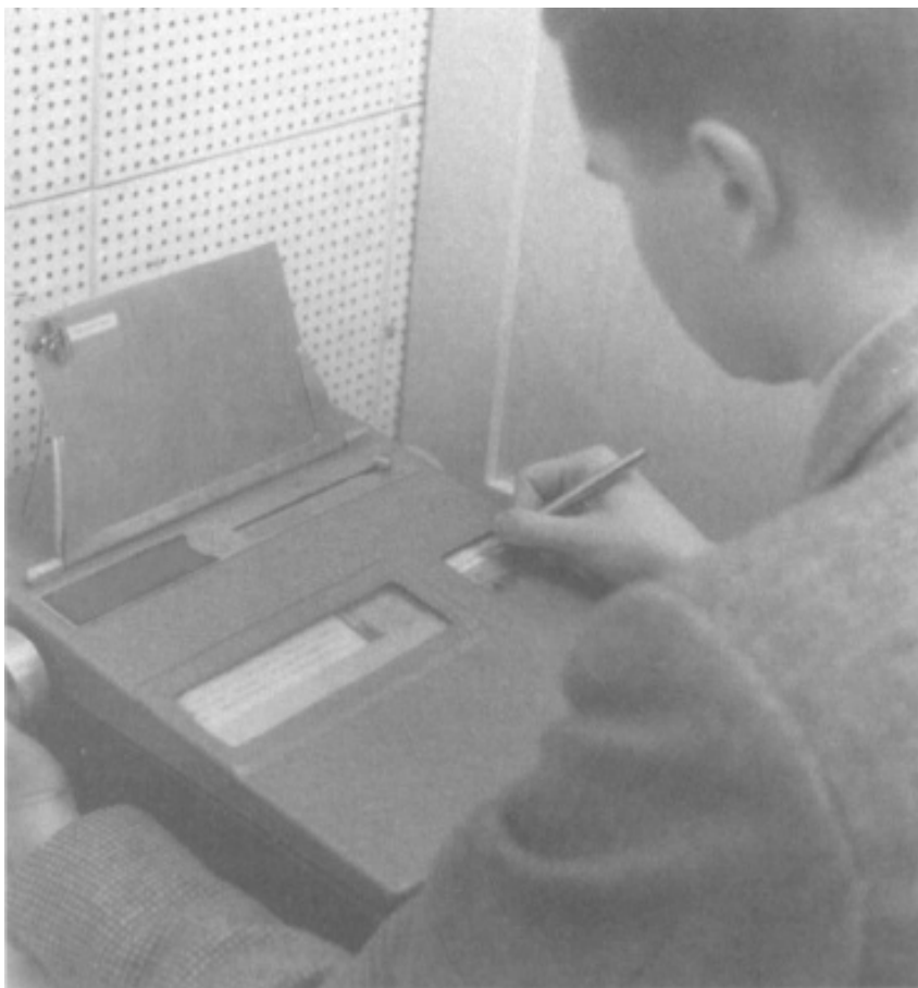
FIGURE 5. A machine similar to that in Figure 4 . Material appears in the window at the left. The student is writing his response on a strip of paper exposed through the small window at the right. By moving a sliding knob at the upper right, he draws a transparent cover over his response and uncovers additional material at the right end of the larger window. This may tell him whether or not his response was correct, often without telling him the correct response. It may also supply additional material. The same movement of the slider uncovers additional space on the strip of paper upon which the student writes a second response if necessary. A further movement of the slider draws a transparent cover over the second response and uncovers the correct response in the large window. A new frame of the material, which is printed on a fan-folded tape, is moved into place by turning the large knob near the student's left hand. The machine cannot be operated until tightly closed and cannot again be opened except by punching a hole in the answer strip. The panel at the rear may hold material to which the program refers.
