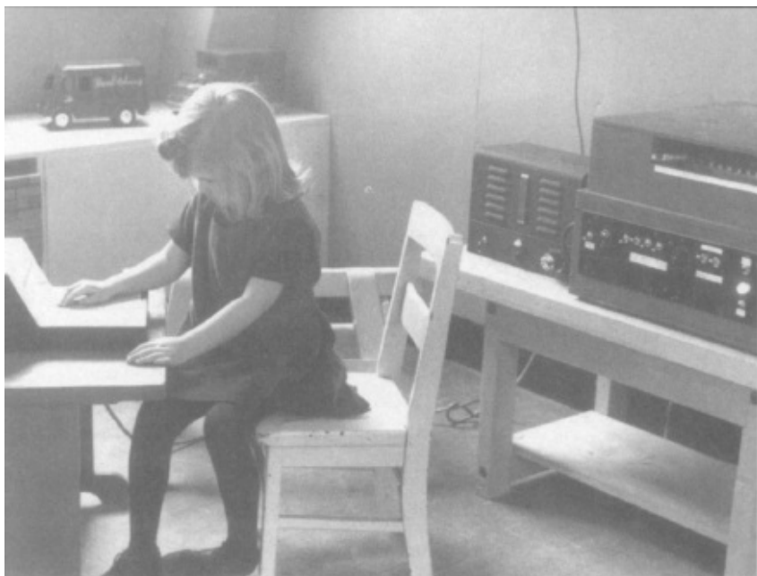
FIGURE 10. A machine to teach “a good sense of rhythm.” The child presses a button in unison with a series of clicks, presented at different speeds and in different patterns. Coincidences are reported by a flashing light. The machine can adjust the tolerance which defines a coincidence.
